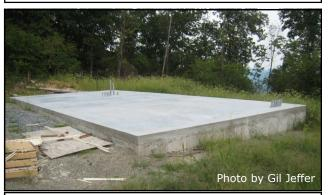
The 20 by 40 foot foundation for the NJIT telescope awaits the next phase of construction.
