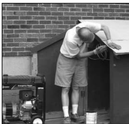
Bill Eberly (MMAS) puts the finishing touches to the shed.
