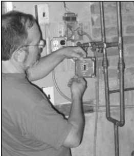
Gill Jeffer installing the emergency switch by the furnace.
